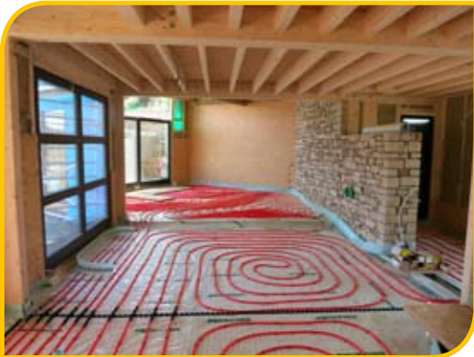
Plancher chauffant
